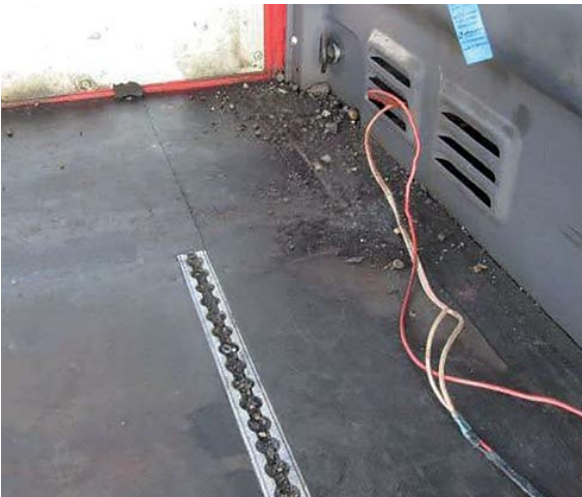
Improper cable wiring by the costumer
